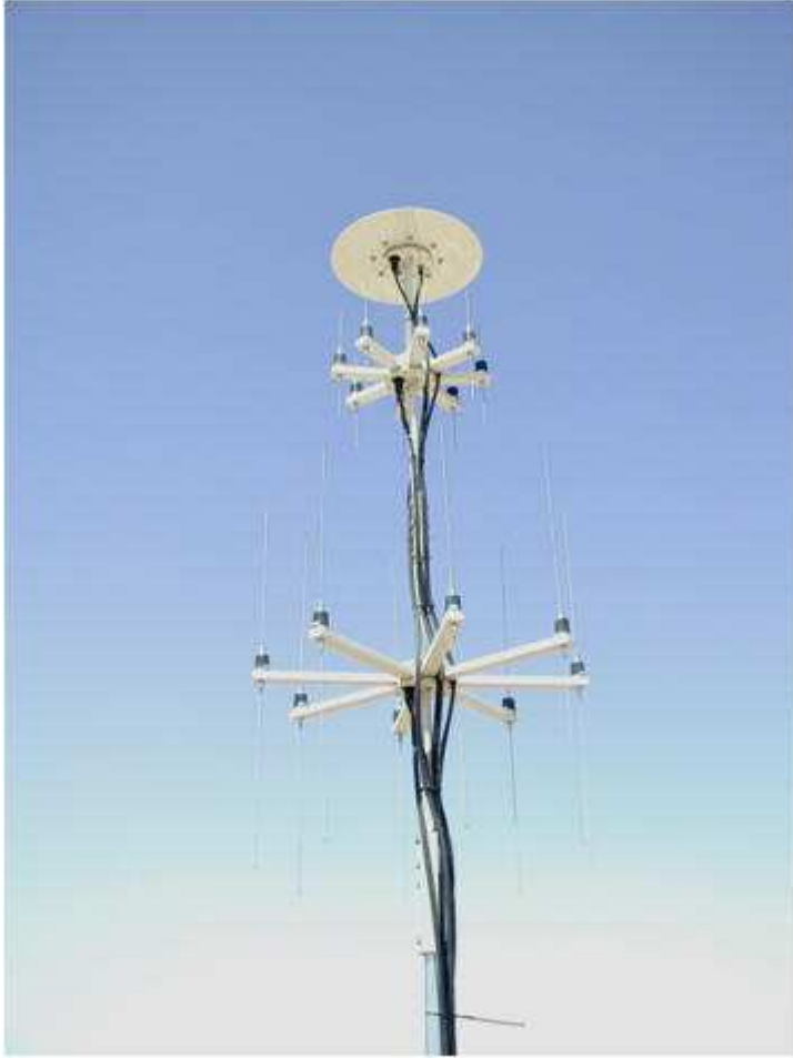
Stack of Three DF Antennas Showing Routing of EPDM Hoses to Lower Two Antennas
